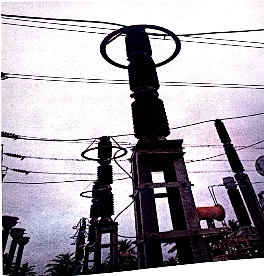
Fig 4.7 Metal oxide surge arrester
