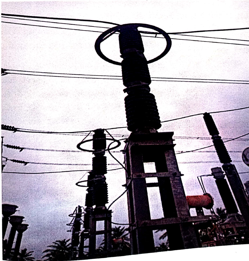
Fig 4.7 Metal oxide surge arrester
