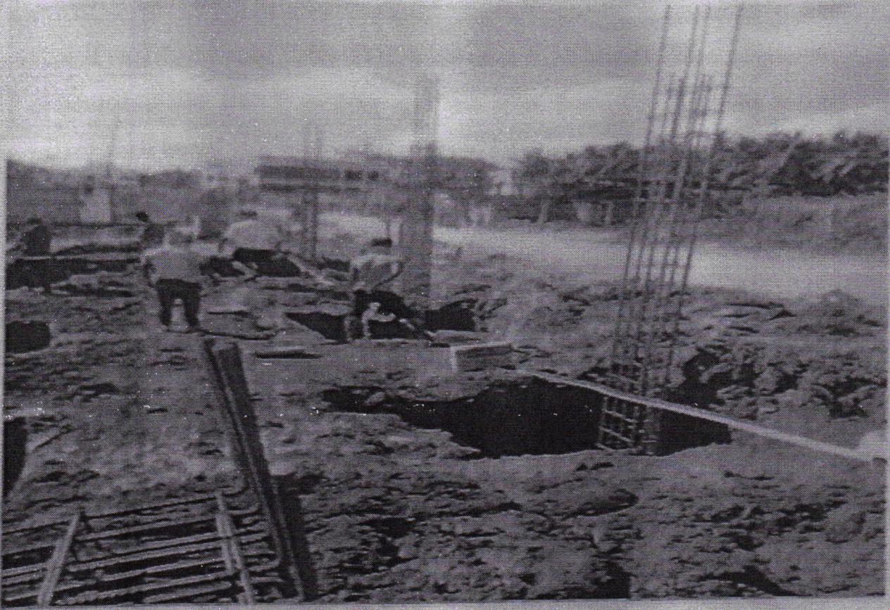
Fig 7 Placating of columns
