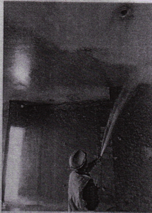
Figure 3.20 : Picture of ceiling plasters curing
