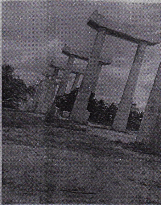
Fig.02: Pier and Pier cap
