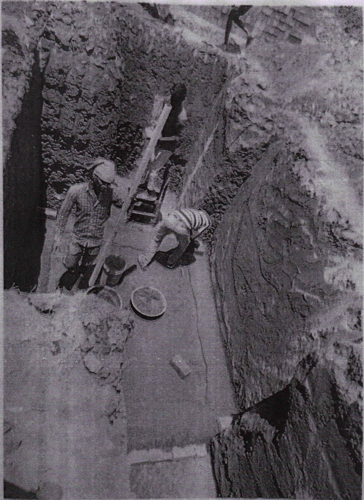
Fig 3.7.3 Laying of foundation
