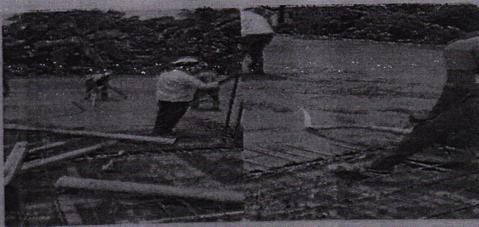
Fig8.3 Needle vibrator
