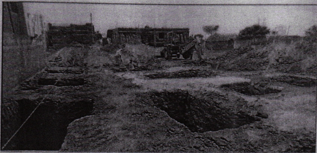
Fig 5.2: Excavation at Site
