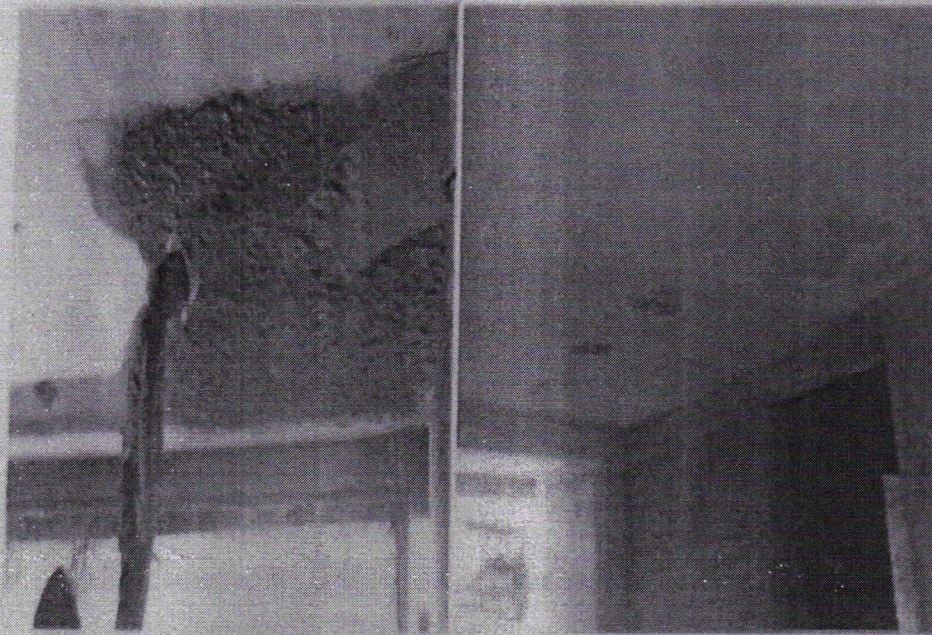
Figure 3.19: Picture of completed first layer plaster
