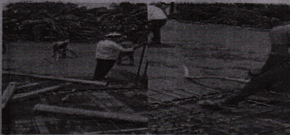
Fig8.3 Needle vibrator
