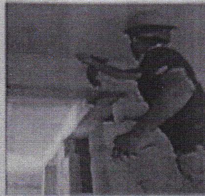
Fig. 8.5.3 Bull marking on ceiling
