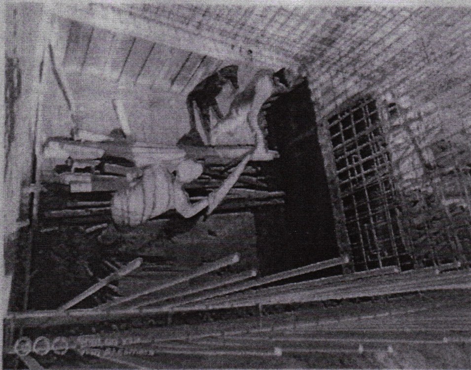
Fig sewage treatment tank , shuttering removing process
