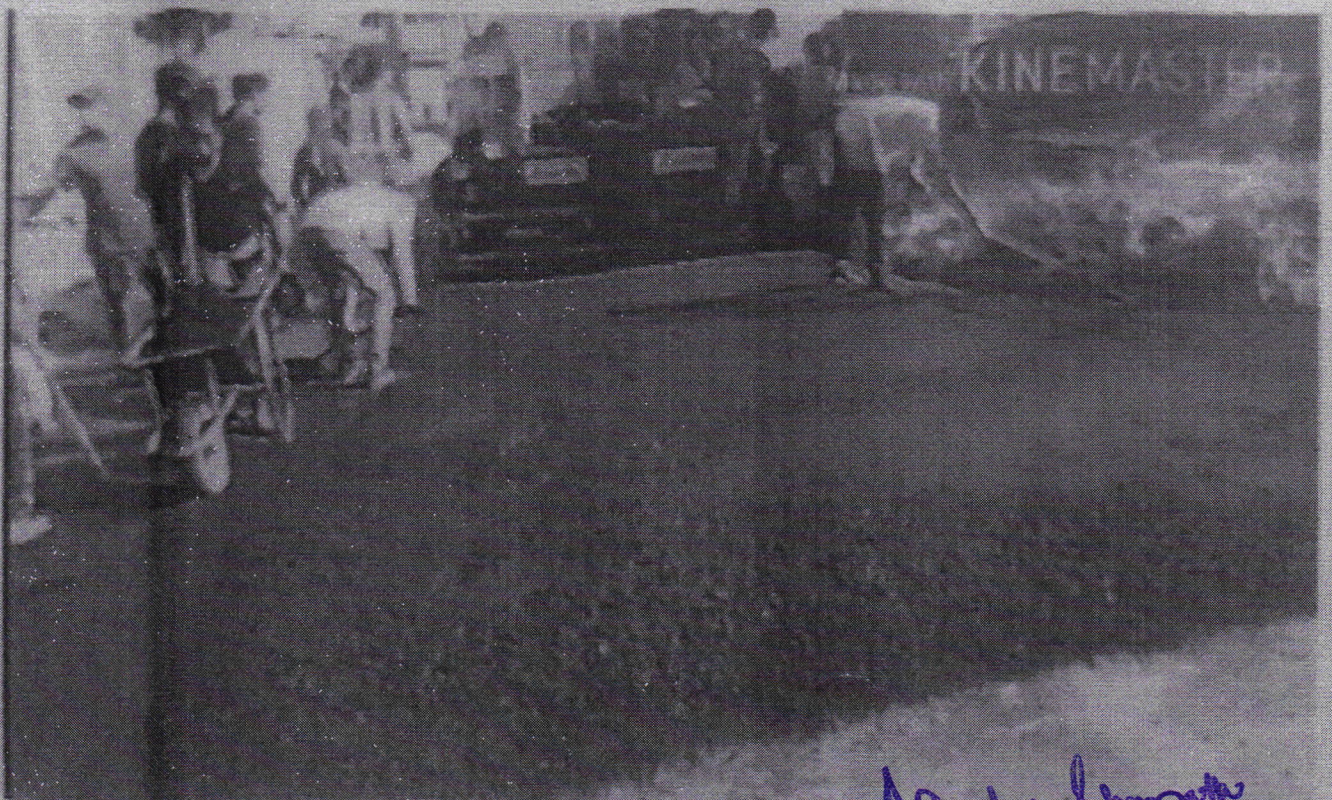
Fig 5.1.3 Placing of premix
