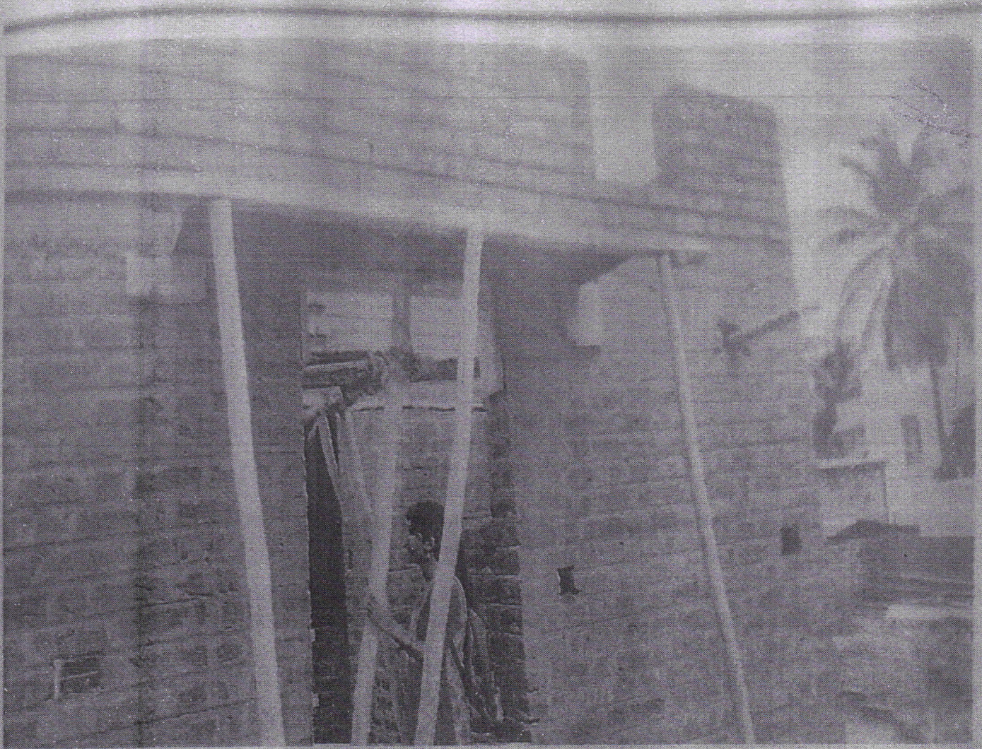
Fig8: Formwork
